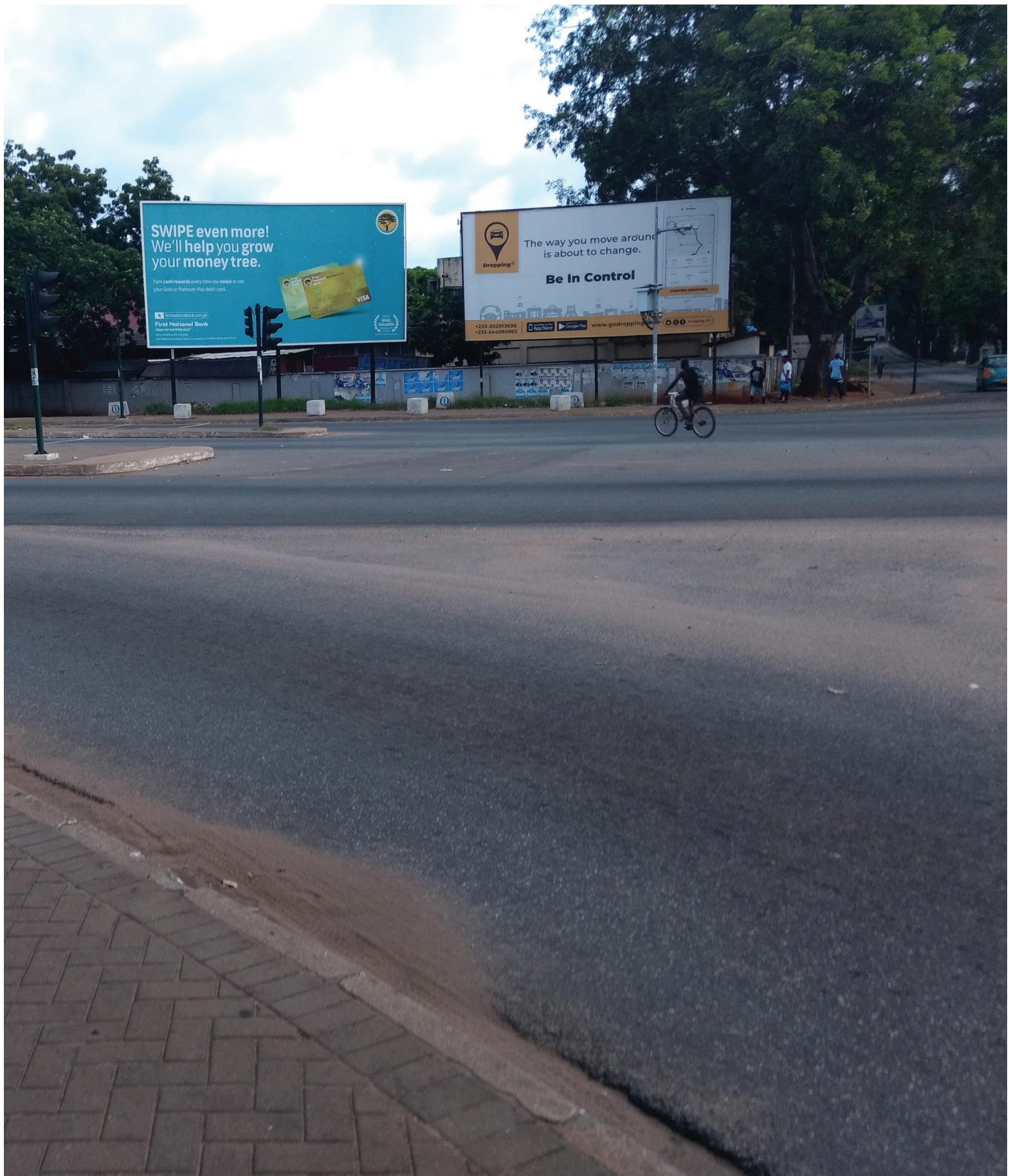
Looking south across Castle Road. The wide corner radius reduces visibility for vehicles and pedestrians, thereby reducing safety.
