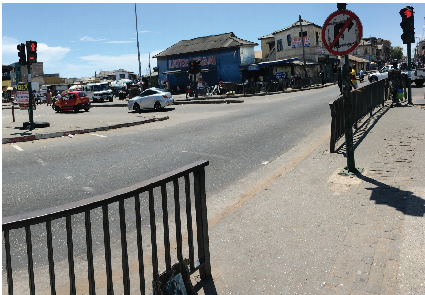
The guardrails cause bottlenecks during periods of peak pedestrian traffic, lengthening the time pedestrians are exposed to vehicular traffic.
